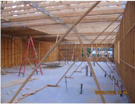
Photo #7: Two of 3 bays w/sheathing with additional bracing
