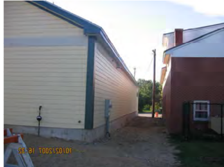
Photo #1: Cement board siding completed on hardware store side Photo #2: Cement board siding completed on alley/back side of new store Photo #3: Cement board siding on gable section completed on RT 2 side
