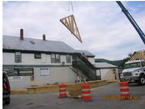
Photo #4: Crane extended over height of hardware store Photo #5: Adding additional bracing to a truss Photo #6: Swinging truss up and over hardware store
