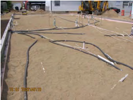
Photo #1: Standing in the kitchen area looking out at conduits for sinks, drains, coolers, etc. Photo #2: Town Water connection (copper pipe on right) next to the central distribution point for water. Photo #3: Conduits for the bathrooms
