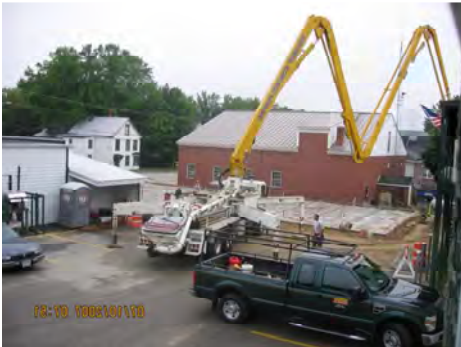
Photo #1: Pump Truck and Boom and spreading concrete
