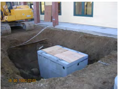
Photo #1: Grease Trap Installation
