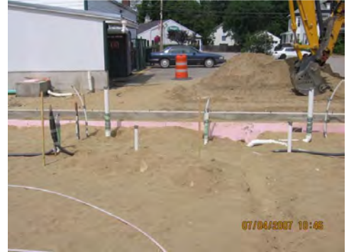
Photo #1: Standing in the kitchen area looking out at conduits for sinks, drains, coolers, etc. Photo #2: Town Water connection (copper pipe on right) next to the central distribution point for water. Photo #3: Conduits for the bathrooms
