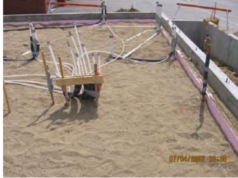
Photo #1: Standing in the kitchen area looking out at conduits for sinks, drains, coolers, etc. Photo #2: Town Water connection (copper pipe on right) next to the central distribution point for water. Photo #3: Conduits for the bathrooms
