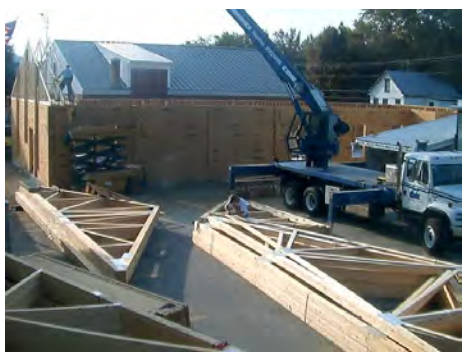
Photo #10: Seating area with sheathing and truss work completed
