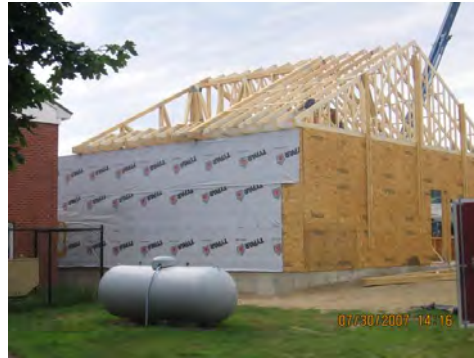
Photo #2: Truss for one of the bays
