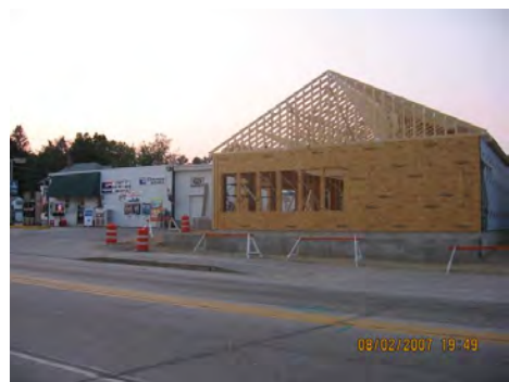
Photo #10: Seating area with sheathing and truss work completed
