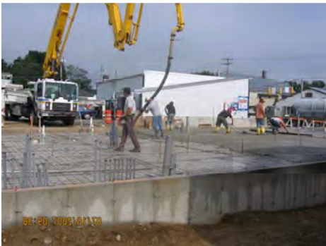
Photo #4: Side view of pouring columns
