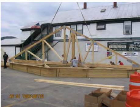
Photo #4: Crane extended over height of hardware store Photo #5: Adding additional bracing to a truss Photo #6: Swinging truss up and over hardware store
