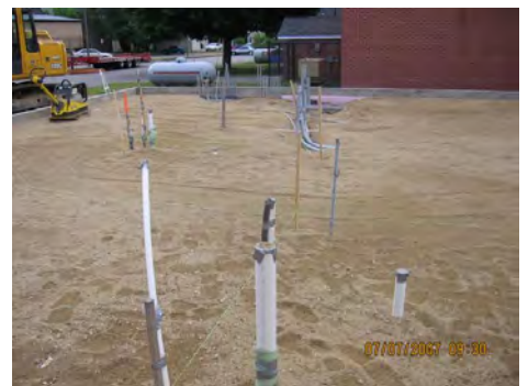
Photo #1: Standing in the kitchen area looking out at conduits for sinks, drains, coolers, etc. Photo #2: Town Water connection (copper pipe on right) next to the central distribution point for water. Photo #3: Conduits for the bathrooms
