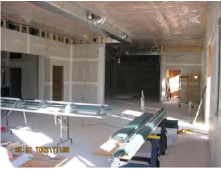
Photo #4: Insulation and sheetrock work almost complete Photo #5: View of Kitchen and seating area Photo #6: Electrical panels continuing to grow
