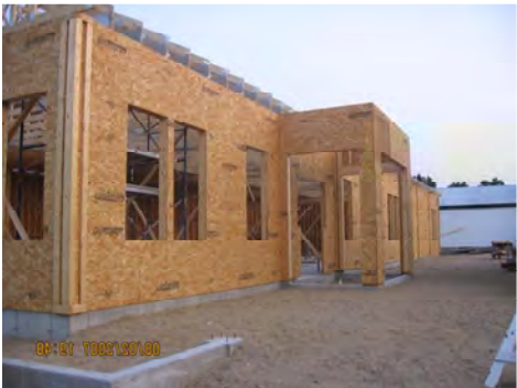
Photo #10: Seating area with sheathing and truss work completed
